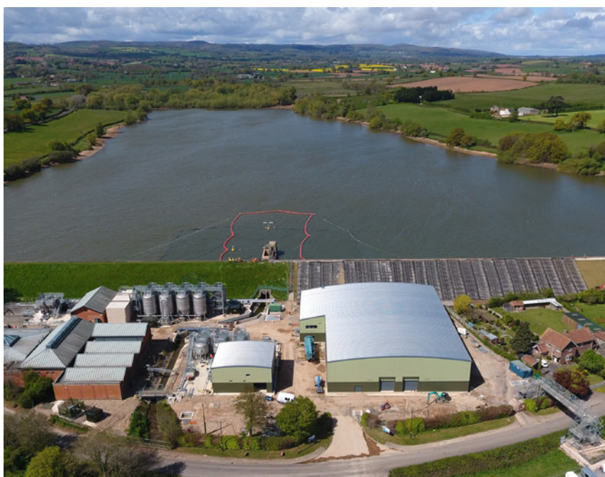
Refurbishment at Durleigh water treatment works, near Bridgwater
