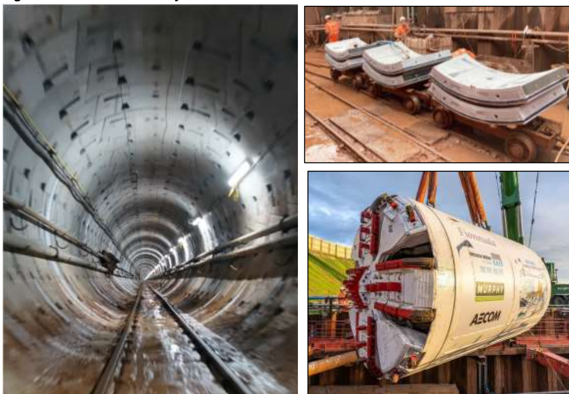
Figure 13: North Bristol – Trym sewer under construction
