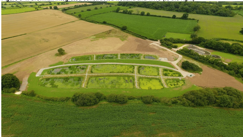
Figure 3-4: Cromhall integrated constructed wetland and WRC (to the right)
