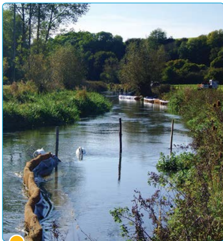
River restoration at East Chisenbury
