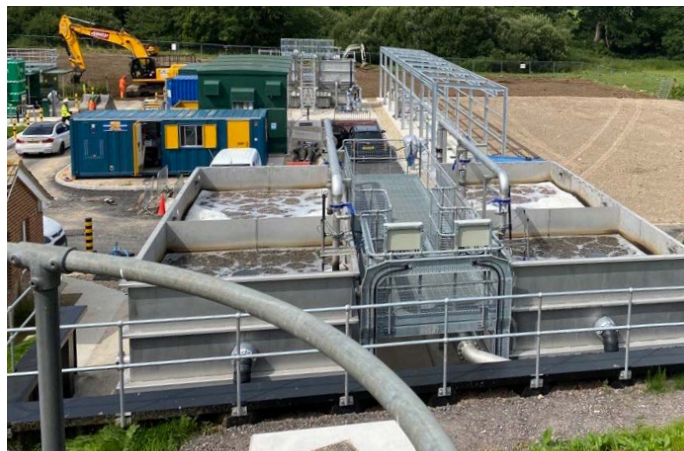
Corfe Castle WRC improvements during construction - July 21. New UV plant in the background, with improved secondary treatment in the foreground
