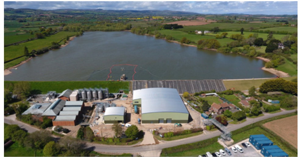
Aerial view of Durleigh water treatment centre improvements
