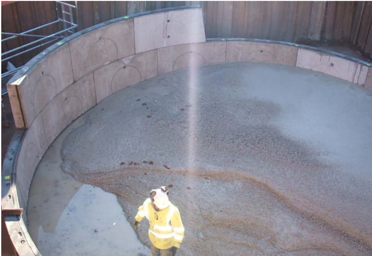
Figure 5-3: Construction of tank 1 (2011)
