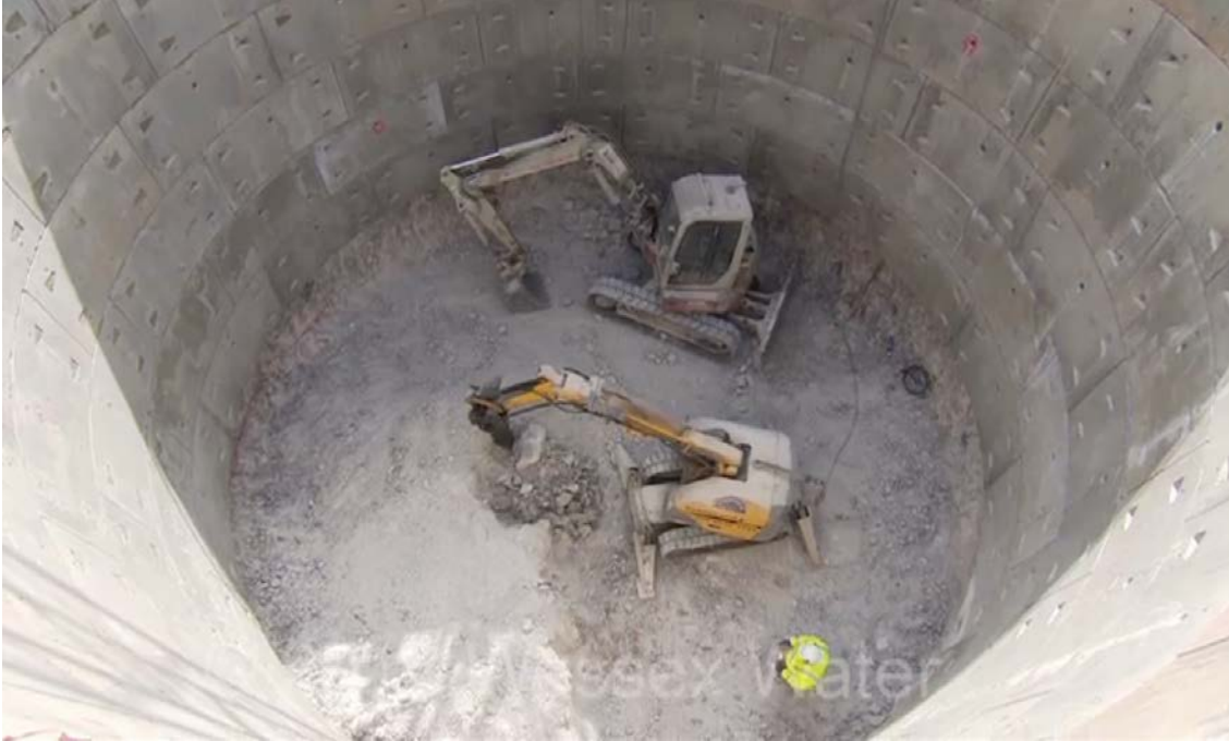
Figure 5-4: Construction of tank 2 (2015/16)
