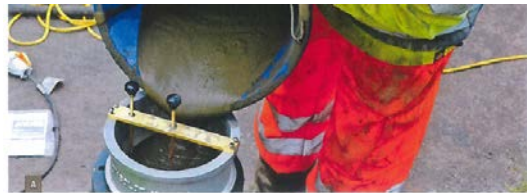
Figure 3-5: Extract from Trenchless International magazine showing our innovative approach
