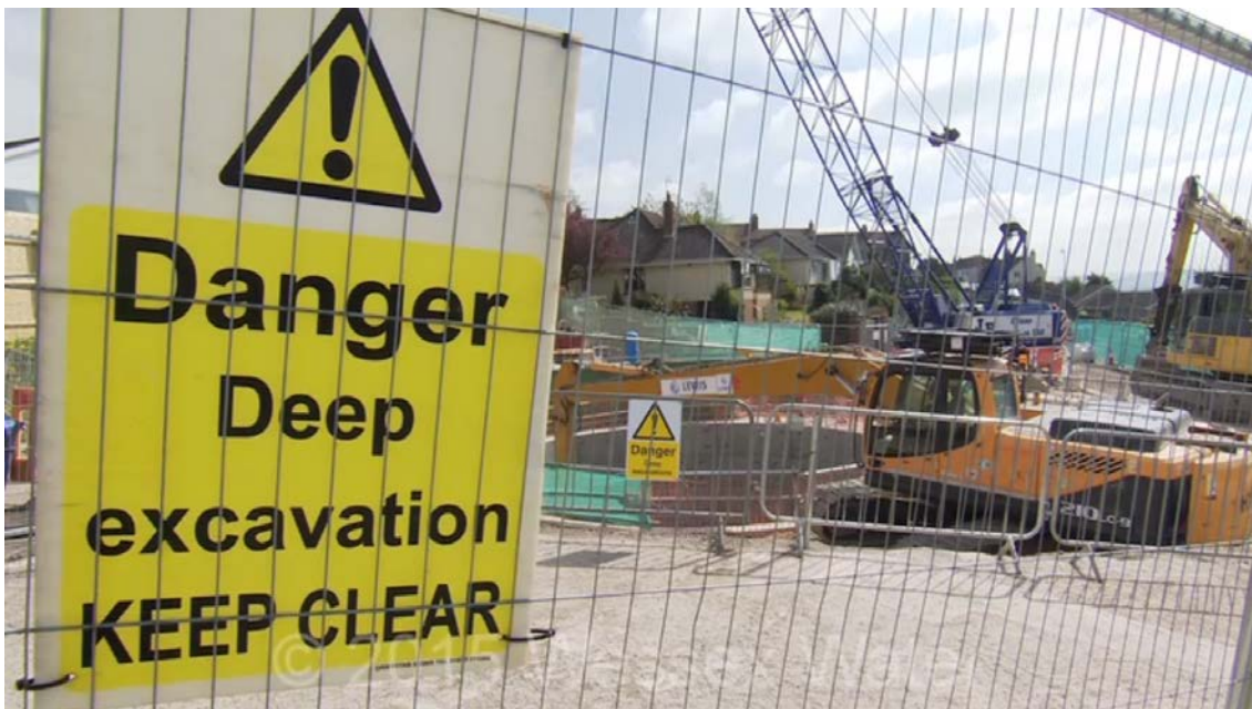
Figure 5-5: Construction of tank 2 in a busy road
